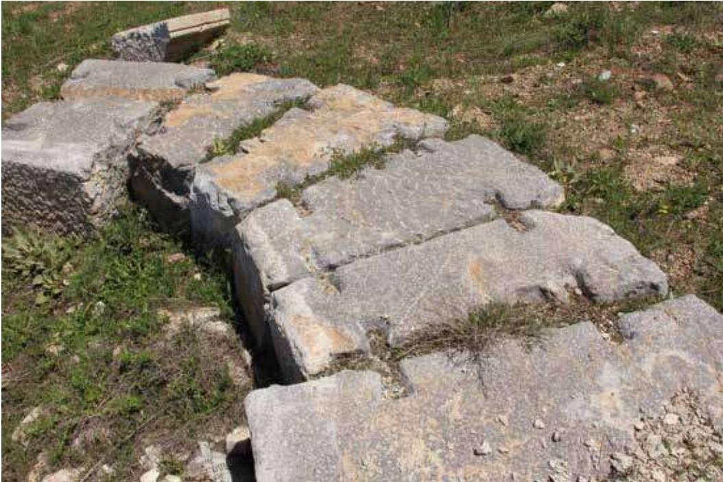
Őek. 27: Pisidia Antiokheia'daki Kuzey Bazilika'nın kırlangı kuyru u krampları tekniđi ile birleŐtirilmiŐ taŐ bloklardan yapılmıŐ stylobat (Fotoğraf: B. Stanisławski) Fig. 27: The base of the apse wall built of stone blocks joined by the so-called swallowtail cramps technique of the Northern Basilica in Antioch in Pisidia (Photograph: B. Stanisławski)
