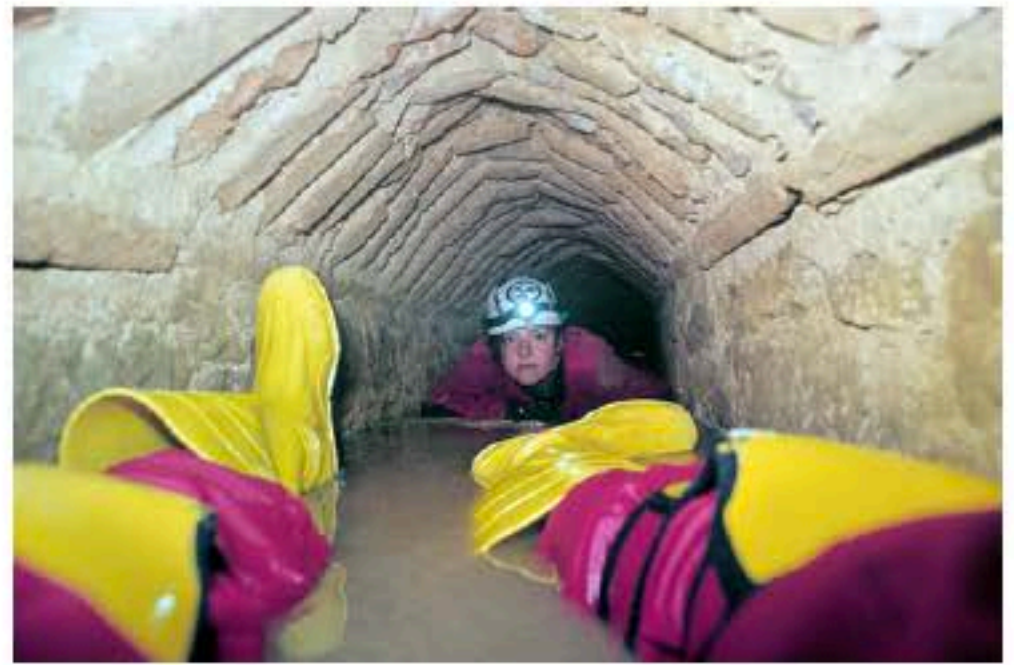
Fig. 13: big Cistern Tunnel (photo Metin Albukrek).
